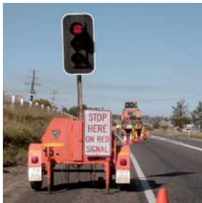
Temporary traffic lights in place. Stop here on red signal.
